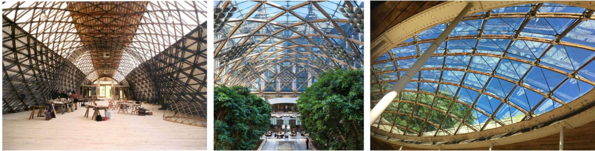
Figure 3: Examples of contemporary timber gridshell structures: (left) Downland Gridshell, (centre) Portcullis House Gridshell and (right) Chiddingstone Orangery Gridshell (Pictures by Edward Culling Architects, Nathaniel Noir and Peter Hulbert Chartered Architect).
